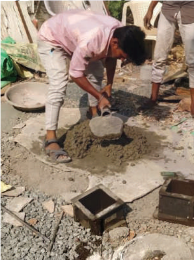
Figure 7.2: Mixing the concrete
