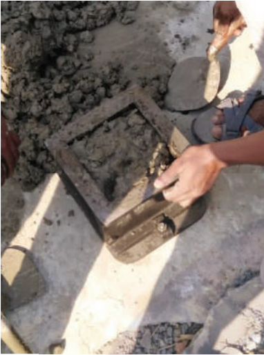
Figure 7.3: Filling the concrete in mould
