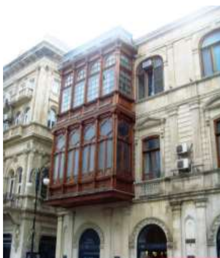
Picture 10: Rented apartment house of Zakiyeva, on the street A.Aliyeva, 3
