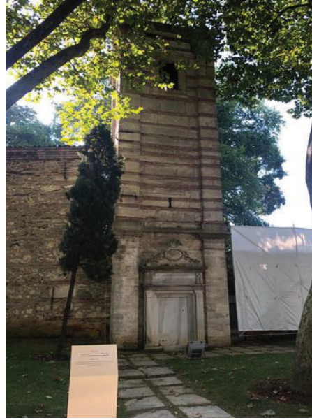
Figure 5. Spirit level view.
